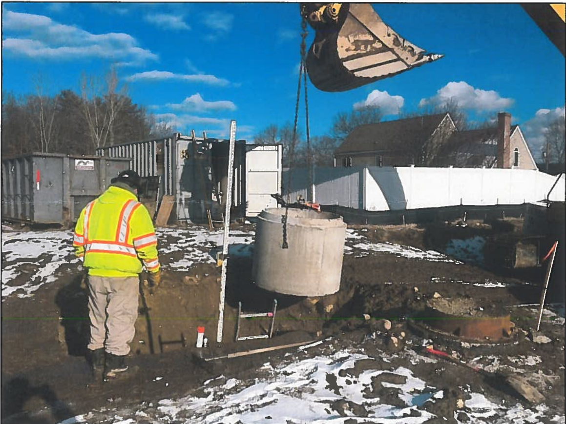
Photo 2: Installation of CB-4.
