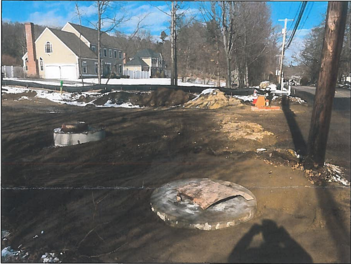
Photo 1: Installed and backfilled CB-1, 2, and DMH-1 on Millstone Drive.
