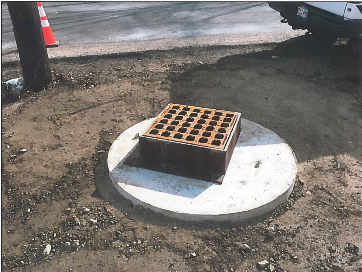
Photo 2: Frame and grate on CB-1.
