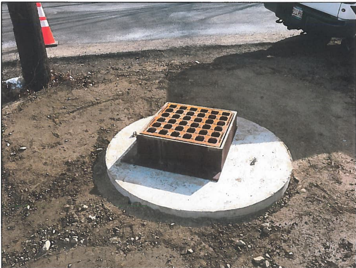
Photo 2: Frame and grate on CB-1.
