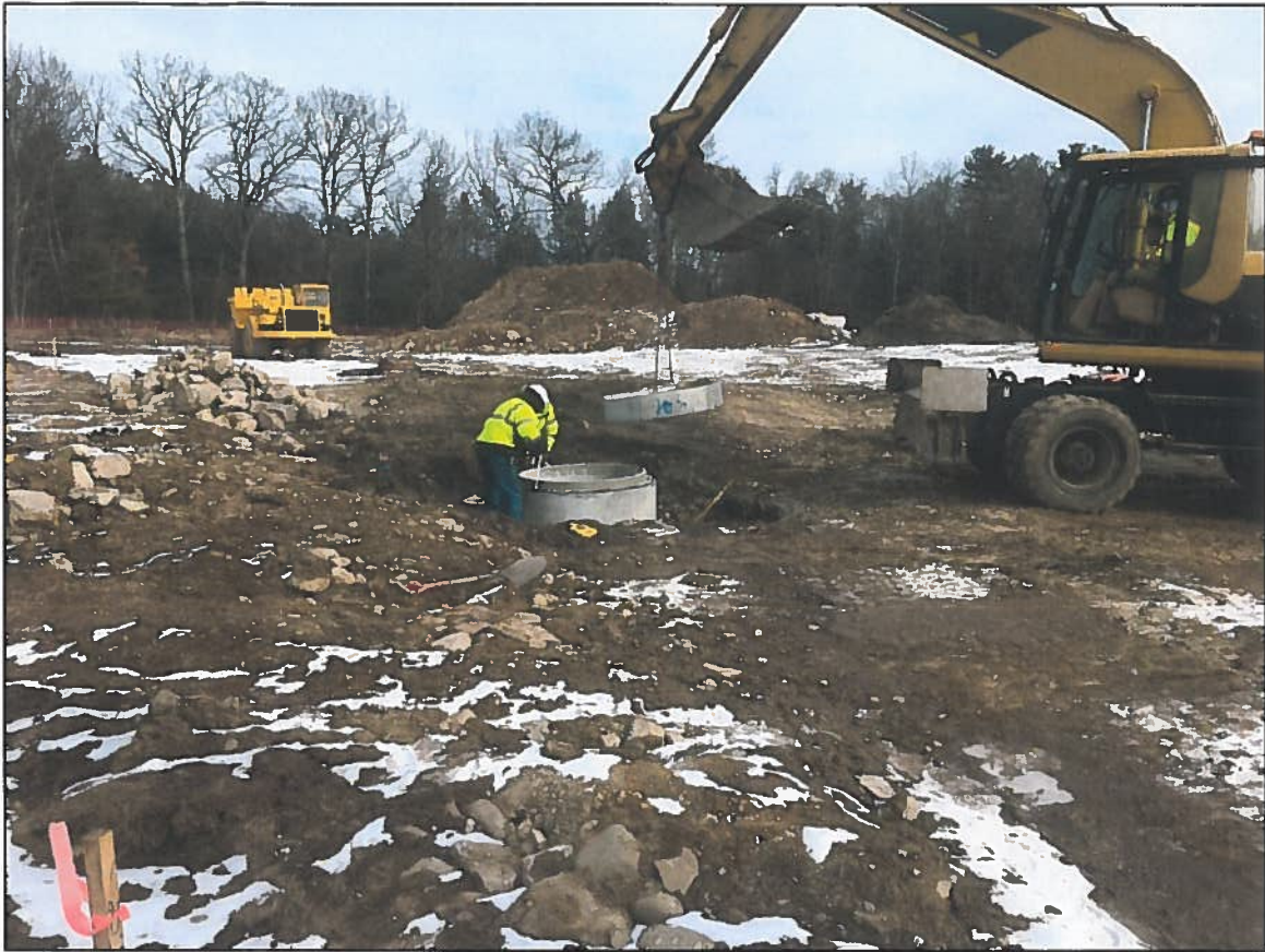
Photo 1: Installation of CB-5 with Kent seal between sections.
