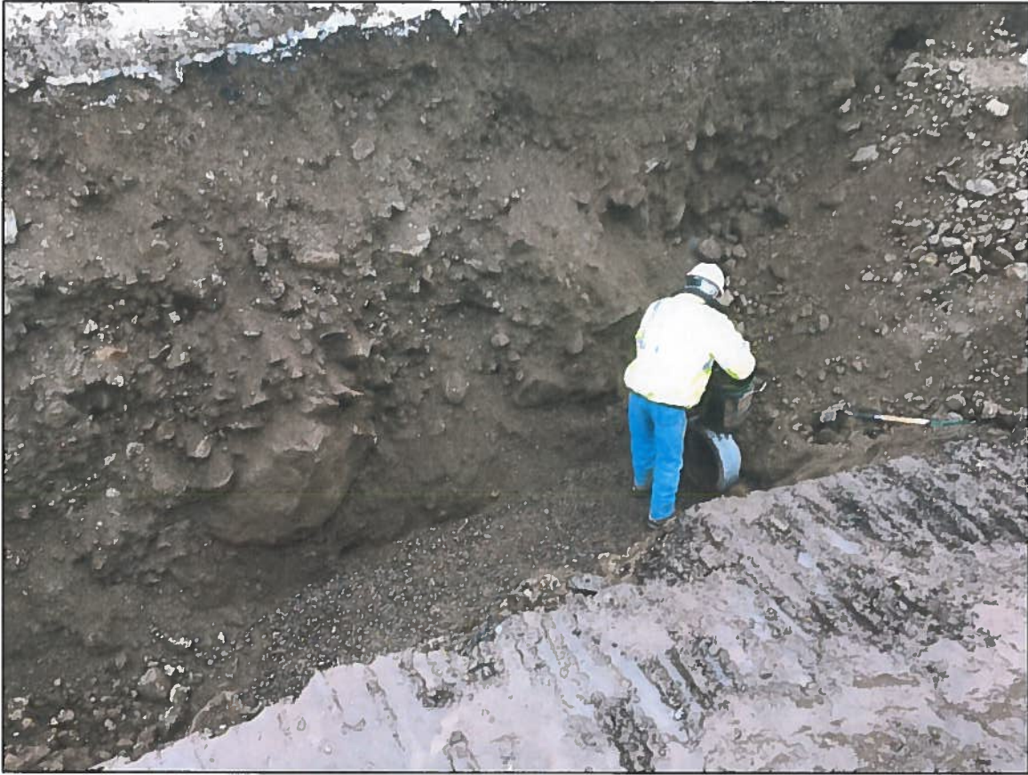
Photo 1: Open drainage pipe trench with installed bed of crushed stone.
