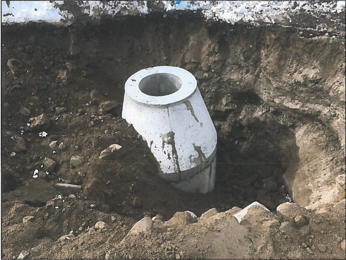
Photo 1: Installed and partially backfilled DMH-7.
