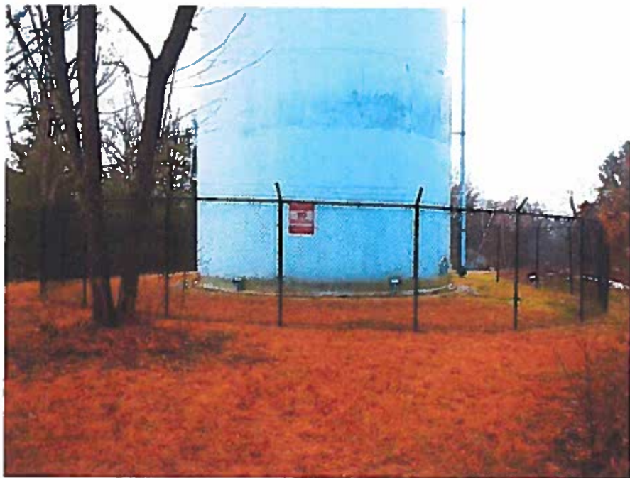
Photo 2: Sample photo illustrating the existing compound where the new T-Mobile equipment pad will be located.
